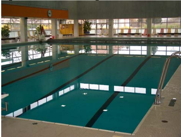
Figure 9 Indoor swimming hall Floridsdorf
