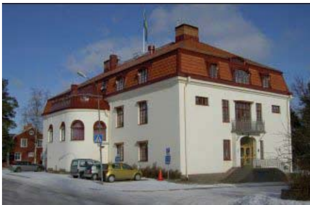
Figure 6 The district courthouse in Hudiksvall
