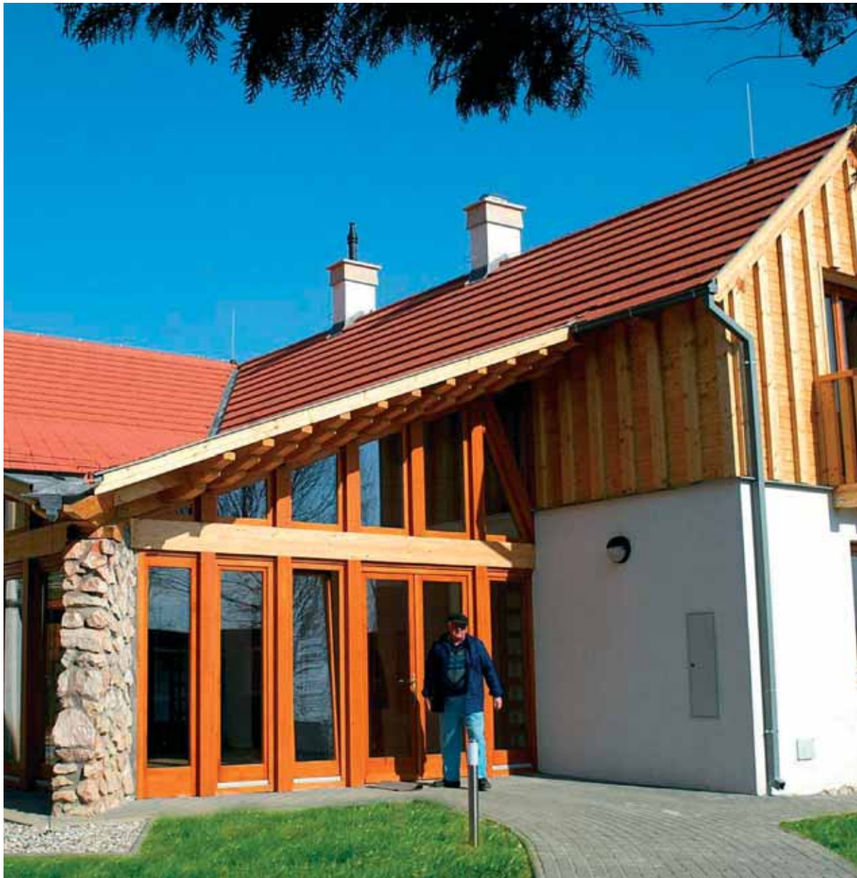
Buildings forming part of the eco-tourism development project
