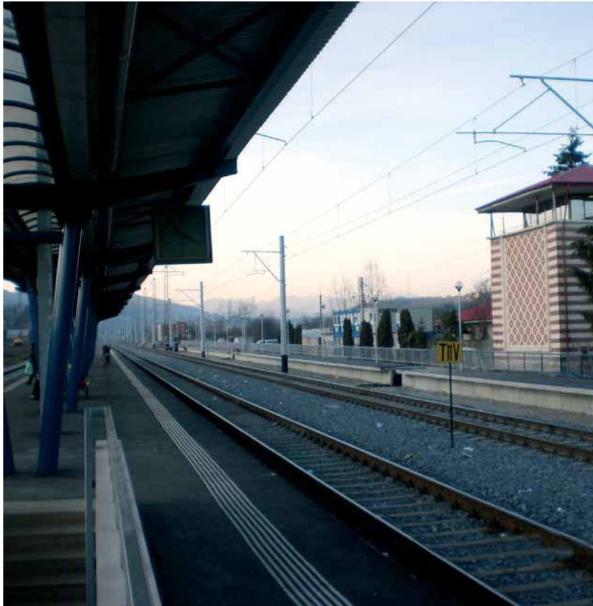
Upgraded rail line connecting people, businesses and goods
