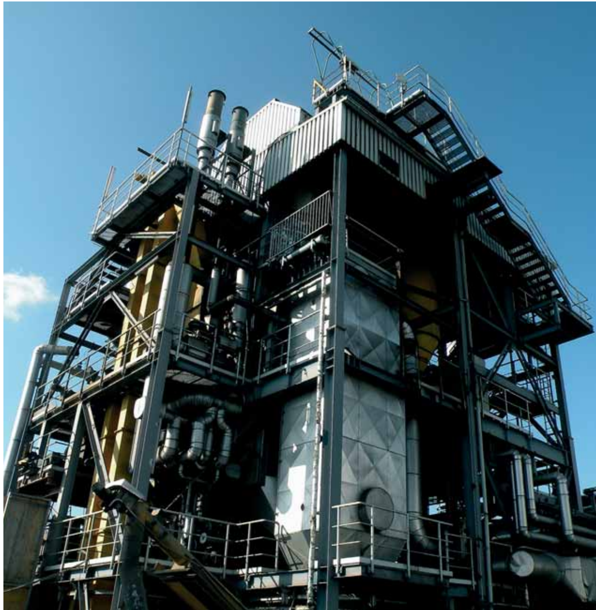
Plant gasifies timber to produce heat, electricity and synthetic diesel fuel
