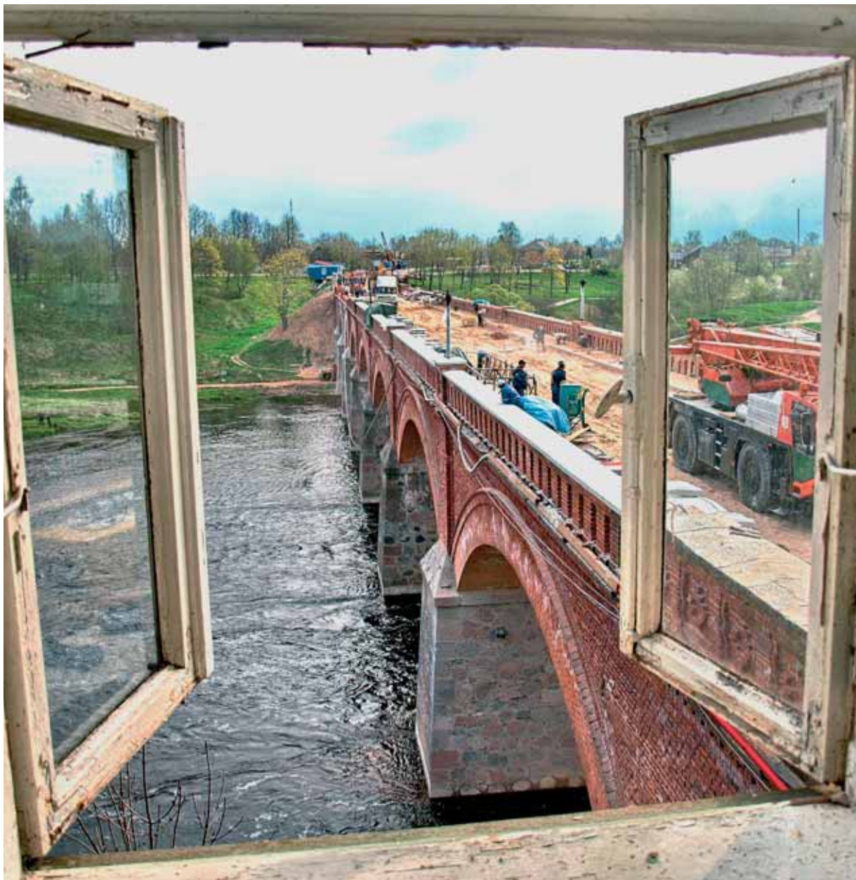
Restoration work in progress on old bridge over the River Venta
